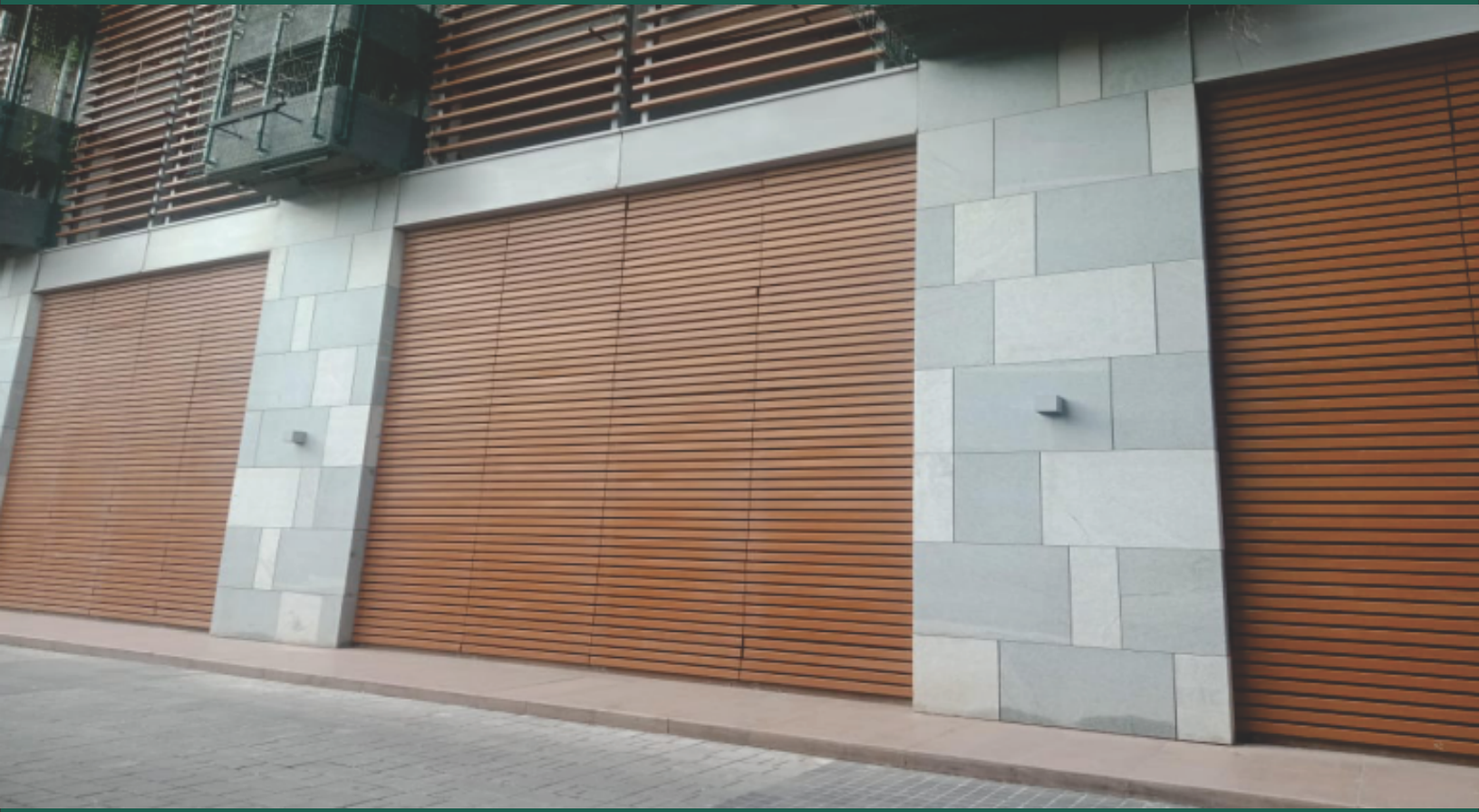
LODHA VENEZIA – STONE CLADDING
