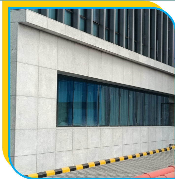
EMERSSION PUNE -STONE CLADDING
